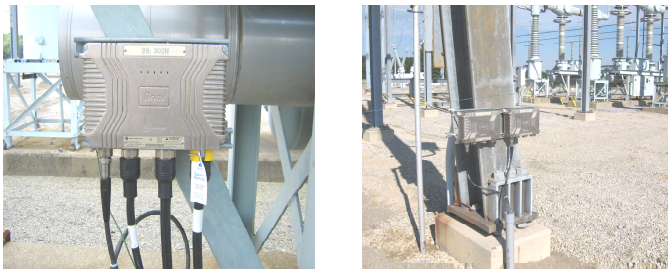
Fig. 7. Merging units and outdoor fiber cables being installed in the switchyard
