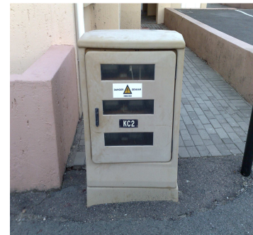
Fig.1 Customers distribution box
