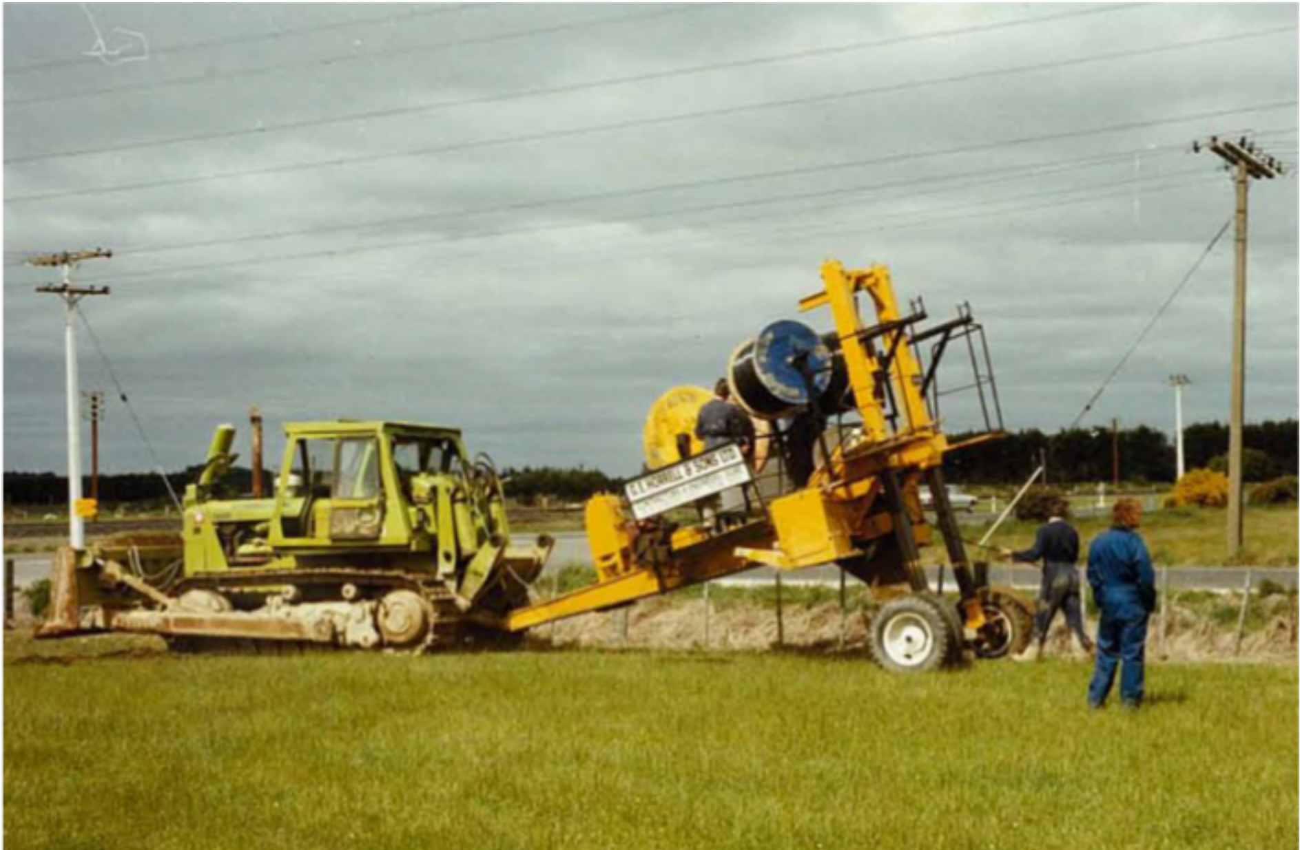
Telecommunications fibre network deployment in Southland
