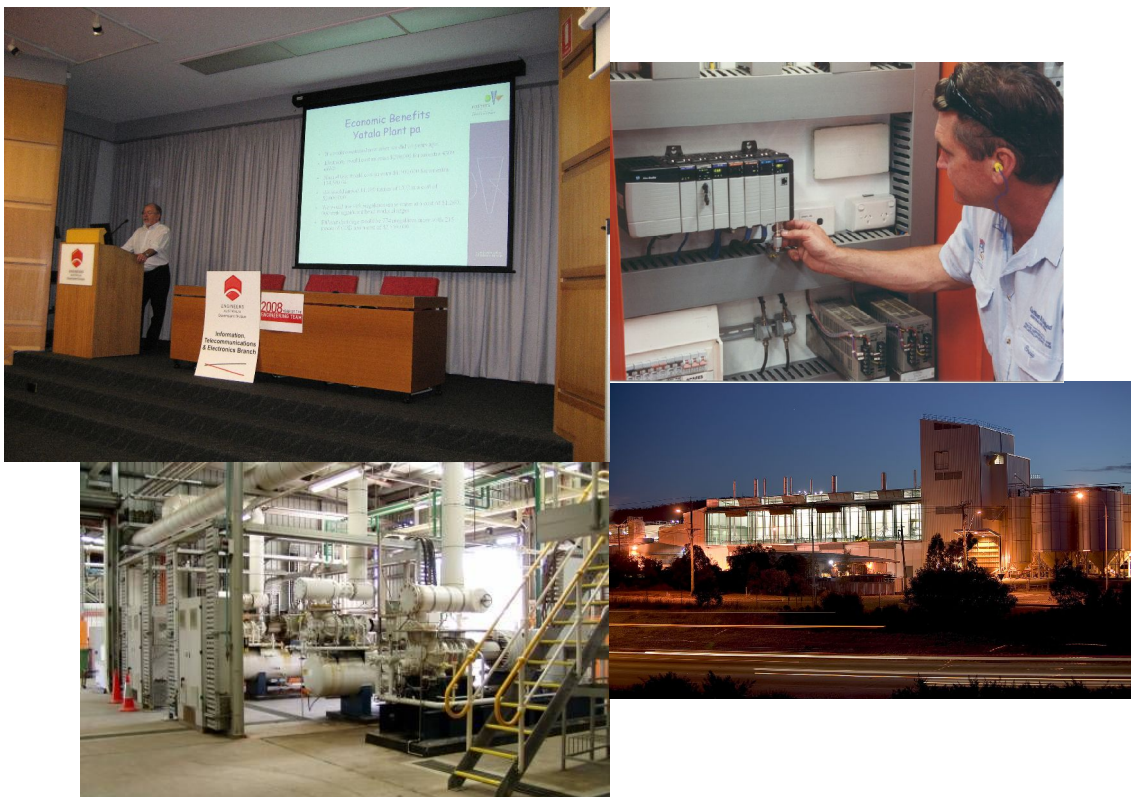
Mr Paul Brodie (top-left) discusses the benefits that Foster's Yatala brewery has seen by embracing automation and technology such as PLCs (top-right) for energy management of key energy consumers including the refrigeration plant (bottom-left) and the Brewhouse (bottom-right). Photos from Paul's presentation are used with kind permission of Fosters Group.
