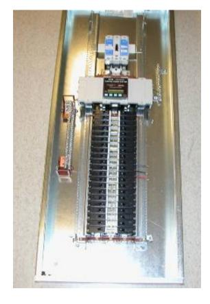
Sidemounted (~14" of twisted conductor)
