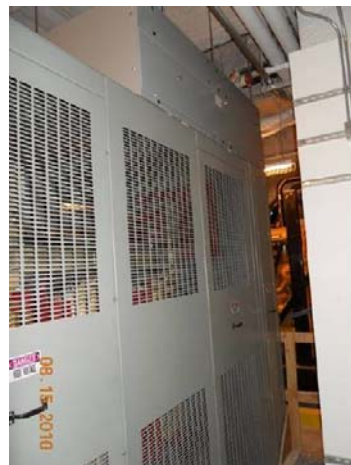
12.47kV snubber mounted horizontally above transformer
