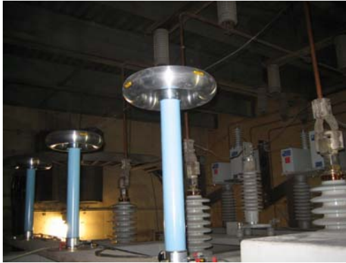
Voltage Dividers Installed at Primary Bushings of Transformer
