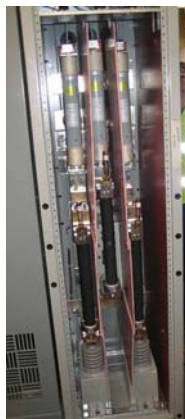
15kV snubber (compact) NEMA1 enclosure
