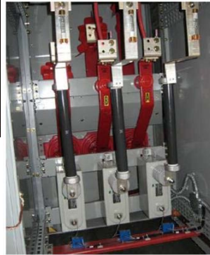
15kV snubber in MV switchgear (switchgear design)
