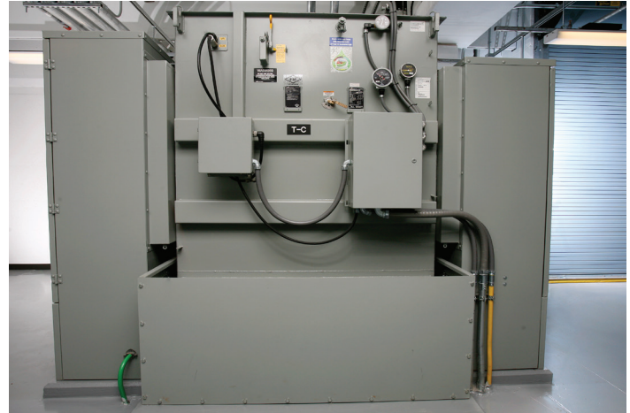
Figure 2. Eaton's Cooper Power series HDC transformer
