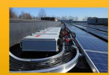
Step 3: Combiner Box connects to the inverter that converts the DC Power to AC Power
