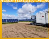
Step 5: The local transformer then sends the stepped-up AC Power to the Main Transformer in the substation where it will be either stepped up again or stepped down depending on the grid
