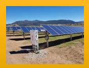
Step 4: The Inverters then send the newly converted AC Power to a local transformer to step up the voltage (usually 34.5kV)
