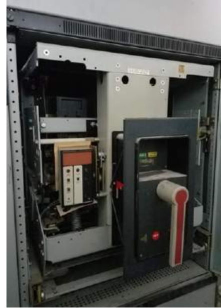
600V Drawout Switchgear with Iron Frame
