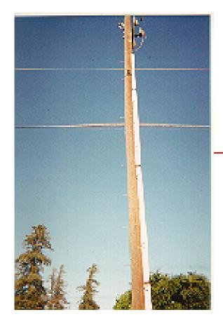
Conductors which extend below the ground line and are generally installed on the surfaces of poles.
