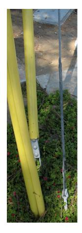
Anchor guys are required to be marked by securely attached markers and in good repair
