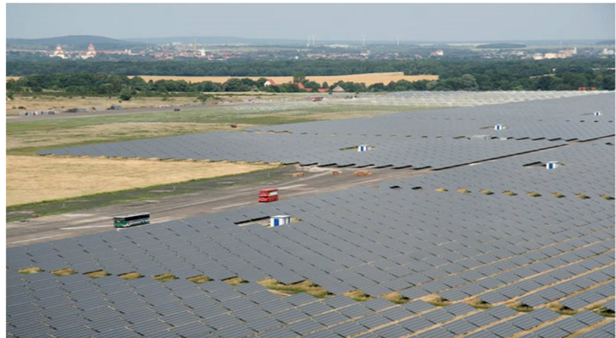
Waldpolenz Solar Park, Germany: 40 MW (generation cost approx $0.30 - $0.40/kWh) (~ 5 times more than fossil fuel generation)
