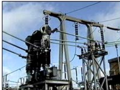
Supplies were affected after the substation fire
