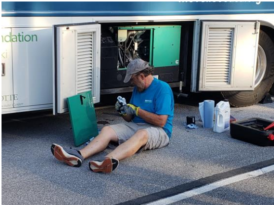
Tim Forest changing generator oil during Hurricane Michael
