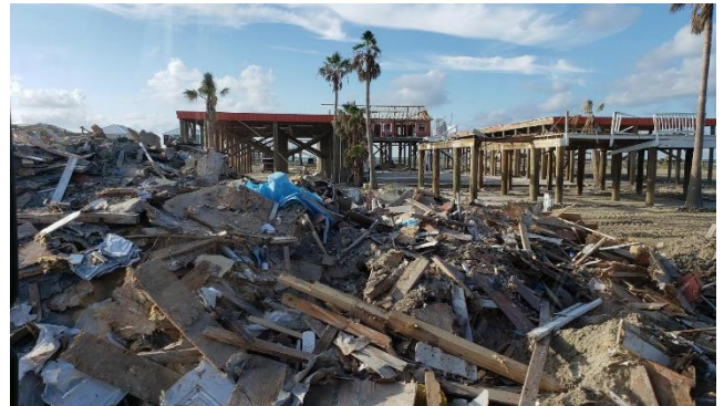
Grand Isle, LA where 80% of structures damaged
