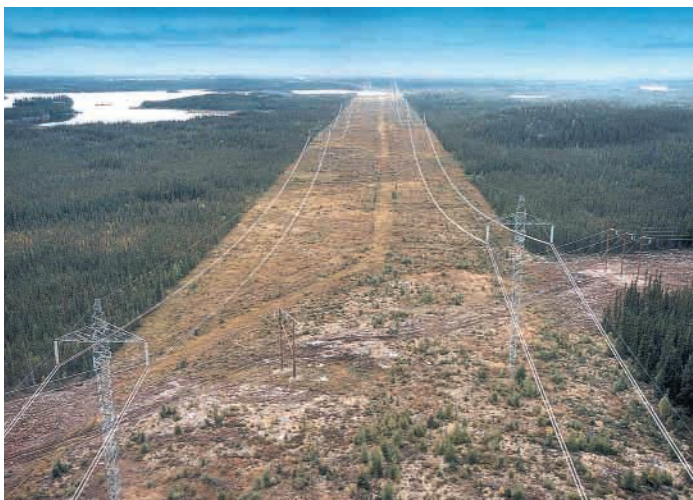
Figure 6: 500 kV HVDC transmission line over the new 230 kV North Central transmission line from Kelsey Generating Station. (Source: Manitoba Hydro).
