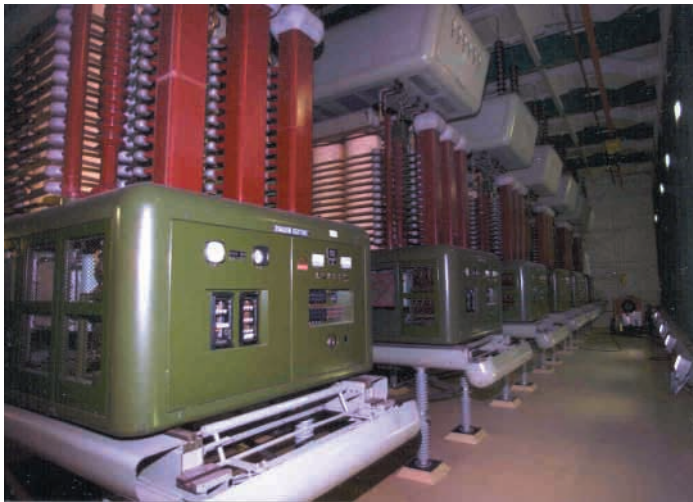
Figure 5: A view of the largest mercury arc rectifier ever built - this type of valve was originally used in the AC-DC conversion stations in the Nelson River DC transmission system. Most of these valves have now been replaced by thyristors. (Source: Manitoba Hydro).
