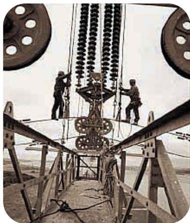
Figure 1: Attachment of 735 kV power lines to insulators with the aid of a crane. The first-ever lines of this type linked the Manic-Outardes generating stations to the metropolitan areas of Québec City and Montréal. Photo courtesy of Hydro-Québec.
