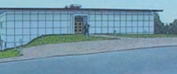
The Clarenville Cable Station, built during the Cold War, was considered a military target because it linked North America with Europe. The station had walls two feet thick to withstand enemy bombs.
