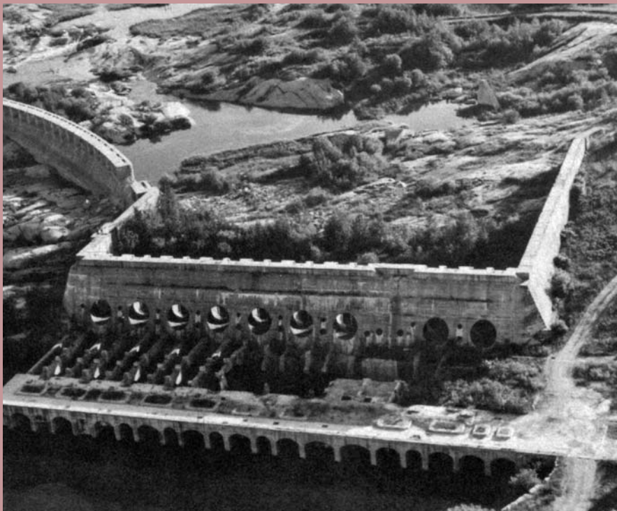
The Pinawa dam—some 65 miles to the northeast of Winnipeg—is located on a natural diversion channel of the Winnipeg River. With the onset of the Great Depression, planned expansion of the Seven Sisters hydroelectric plant was put on hold, giving Pinawa a life extension of 20 years. With modest changes its head was raised from 32 feet to 46 feet, thereby increasing the output from 14MW to 22 MW.
