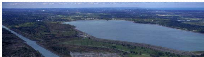
Sir Adam Beck Pumped Generation Station Reservoir (Source: OPG)
