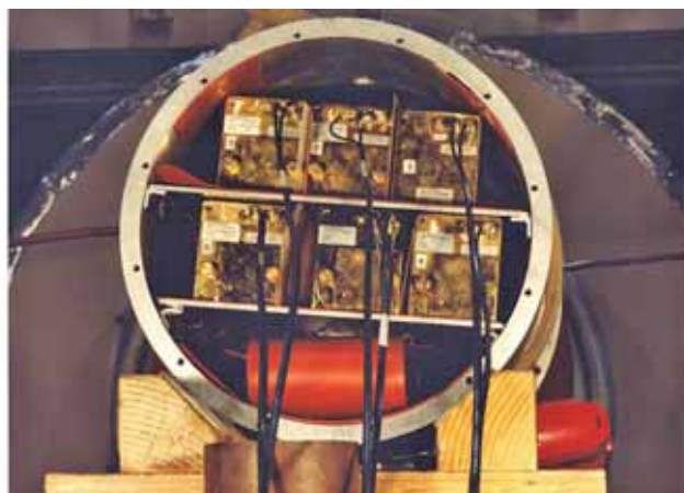
Figure 6. Fiber optic transmitters inside the Instrumentation Barrel.
