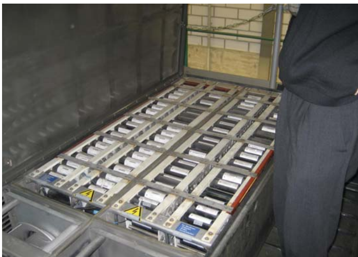
Box with ultracapacitors on the roof of the tram
