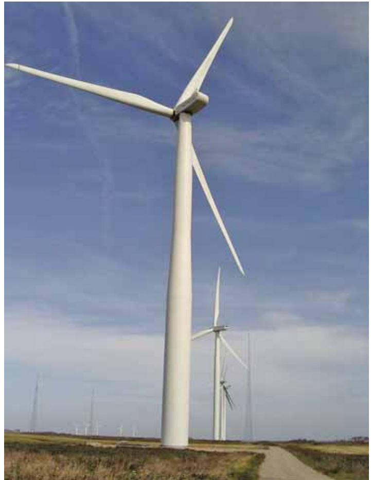
Large Turbine Test Site of the Danish Wind Energy Research. Turbine ratings of 1.5 MW to 4.6 MW under test from various manufacturers
