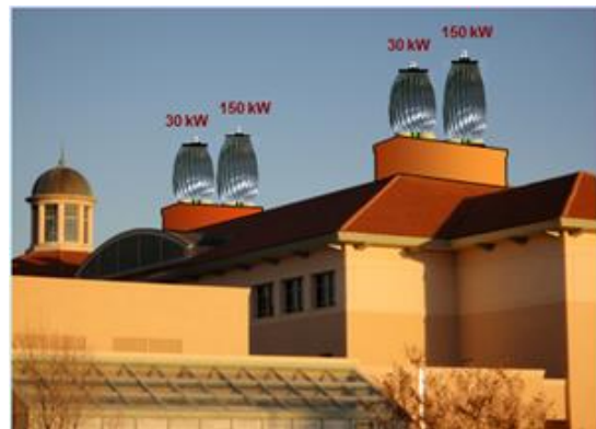
Fig 1: Concept for harvesting energy from building air exhaust systems
