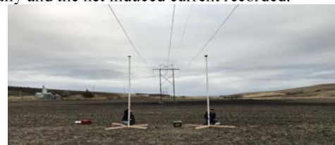
Fig. 3. Photograph of the site with the space potential probe arrangement.
