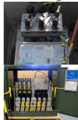
Low profile curbside pedestal enclosure.
