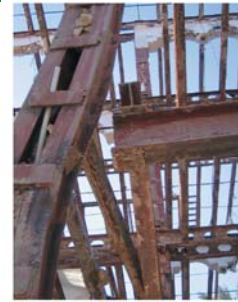
(b) Close-up of the column-beam connection.
