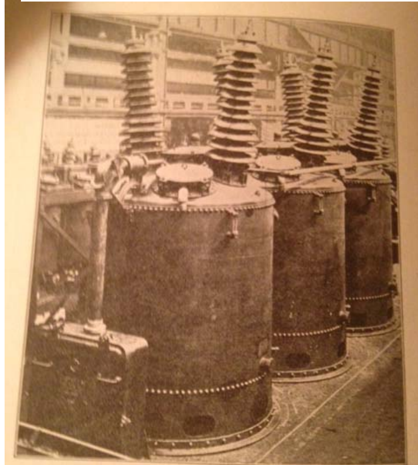
—Westinghouse type “G-2” outdoor oil circuit breaker, 400 135 K.V.
