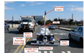
The deployment of the robotic bridge inspection system on the Washington Memorial bridge, Washington DC, USA in 2013.
