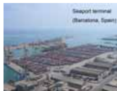
An automated transportation system in a seaport terminal
