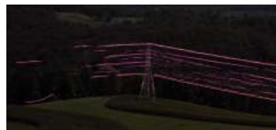
High tension power line detected (pink) at a range of over 750m in a helicopter's forward looking camera.
